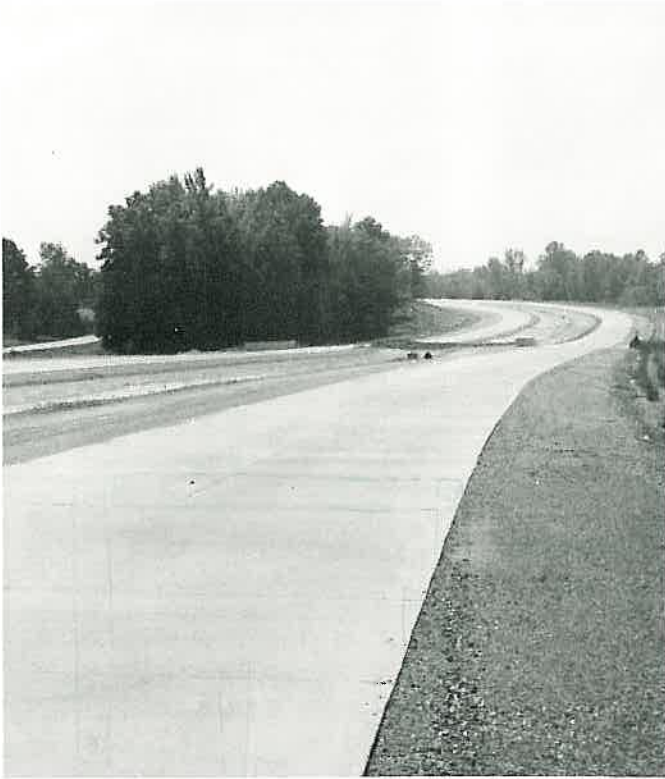
A stretch of the new portion of Highway 65 from Highway 104 to the Pulaski County Line.
